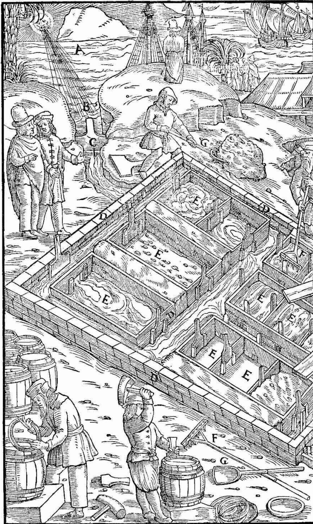
A—SEA. B—POOL. C—GATE. D—TRENCHES. E—SALT BASINS. F—RAKE.
